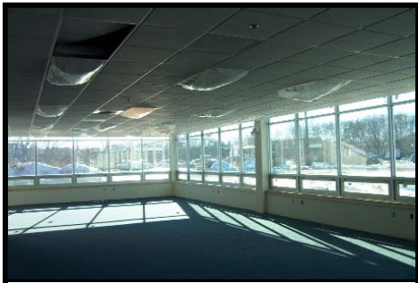
8 Preston Court Interior Photo
